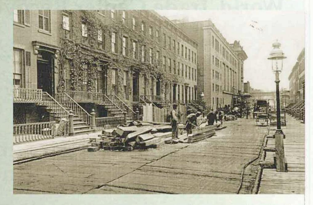
rest of the trench was filled with loose dirt and debris, leaving huge voids below the street surface. Over 75 years, the soil shifted into the voids wreaking havoc on the water mains. The water from the broken mains washed away even more soil, and ultimately the street sank.
